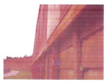
There are no substantial breaks or gaps in the barrier. Given that the current height meets the recommended height of 6m total and is in the correct geographical position then there are no measures that could be undertaken to improve the noise barrier, other than increasing its height. It is therefore fit for purpose and meets the requirements of my original specification.
